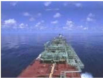
Sendje Ceiba FPSO Bergesen 1x 18V32DF 18'000 running hours
