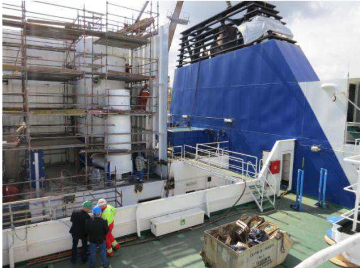
Scrubber installation at Remontowa Shiprepair yard
